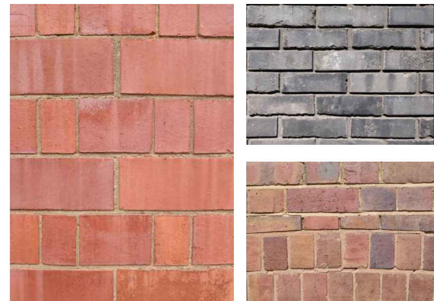
Image: different brick types and bonds found in the Jewellery Quarter
